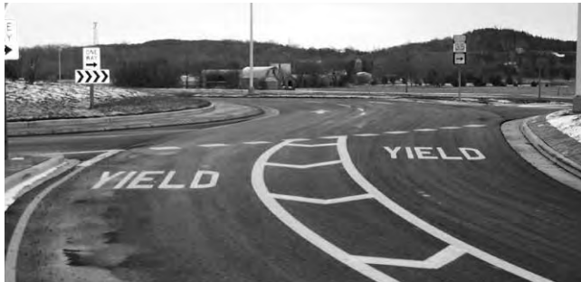
Figure 2.11b: STH 35 and Hanley Road near Hudson
